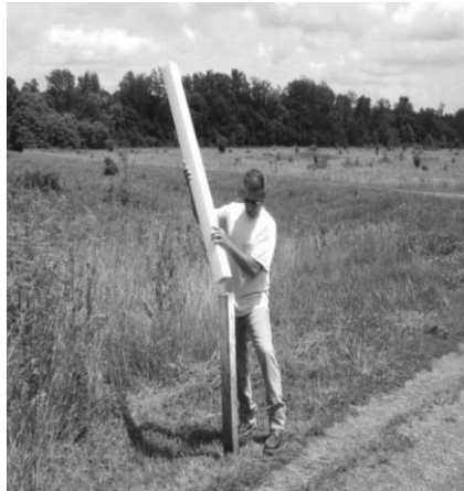
STEP 2 SLIDE VERTICAL SLEEVE Slide vertical en manga
